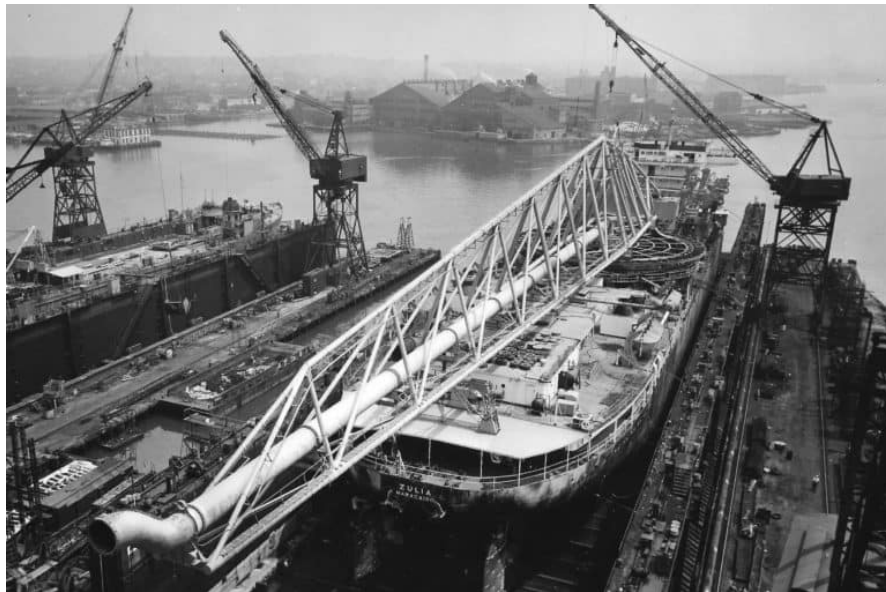
The Zulia was designed and built by Daniel Ludwig in 1959 at the Key Highway shipyard in Baltimore to dredge the Orinoco River. [Photo courtesy: Capt. James McNamara]
